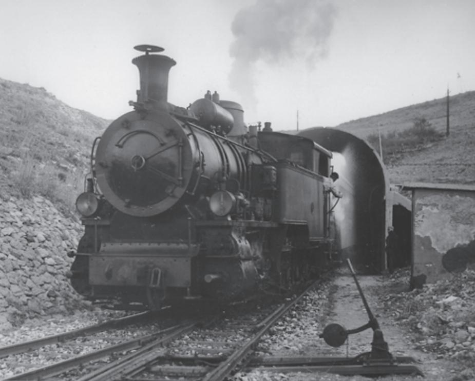
**LEFT AND LOWER** Built in the 1940s, several cement tunnels, like the one depicted here, helped shield the tracks from snow accumulation.
