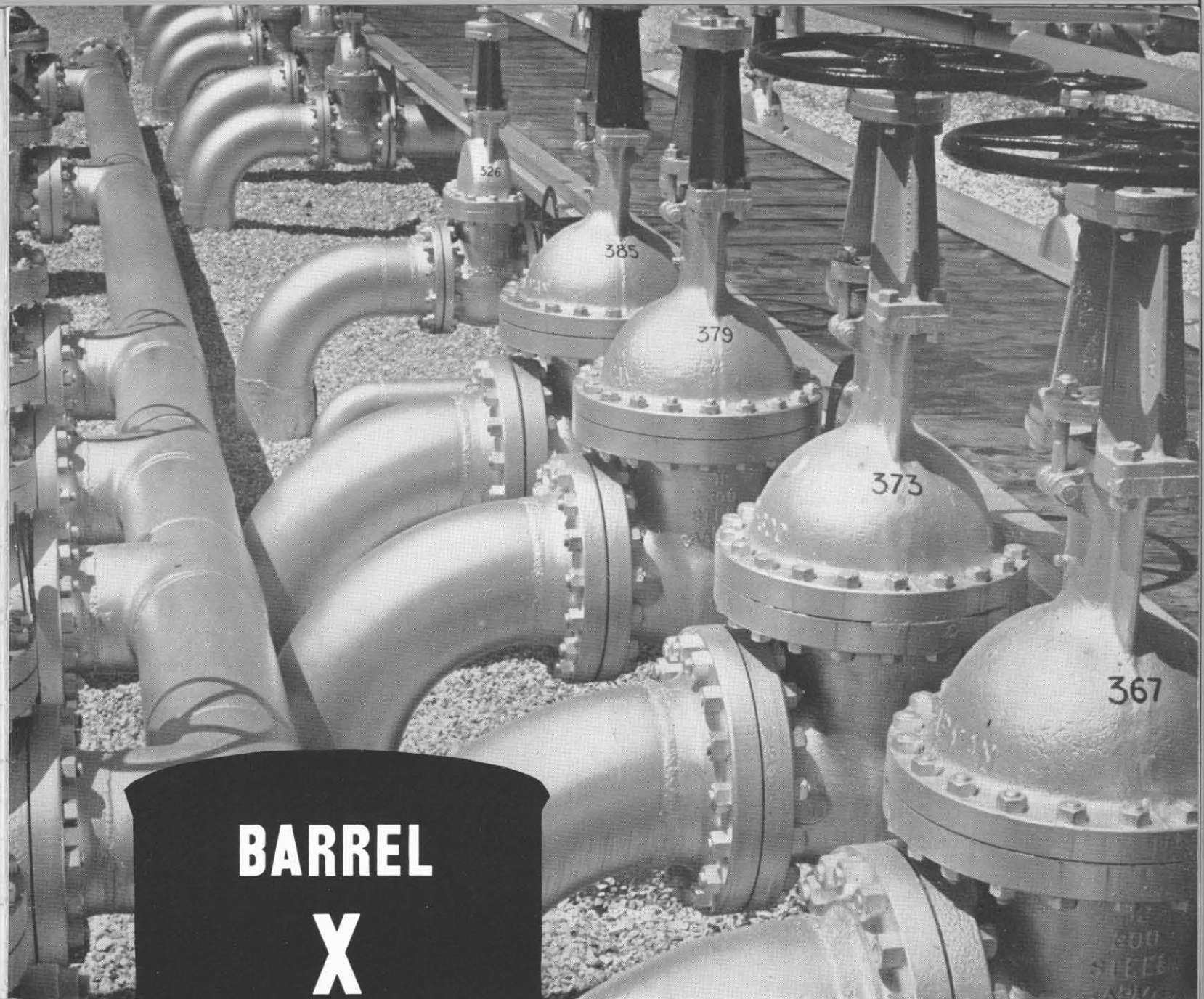
Manifold valves at shore control station of Tapline's terminal at Sidon, Lebanon.
