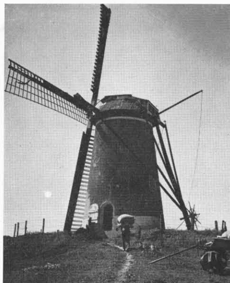
Smock mills are stationary, except for the dome, which is turned to face wind.
