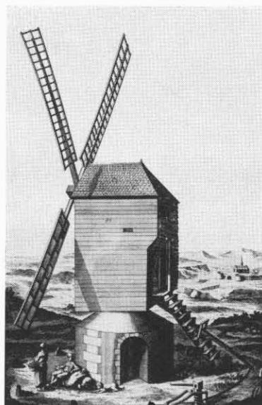
The whole body of this mill rotates on an upright post.
