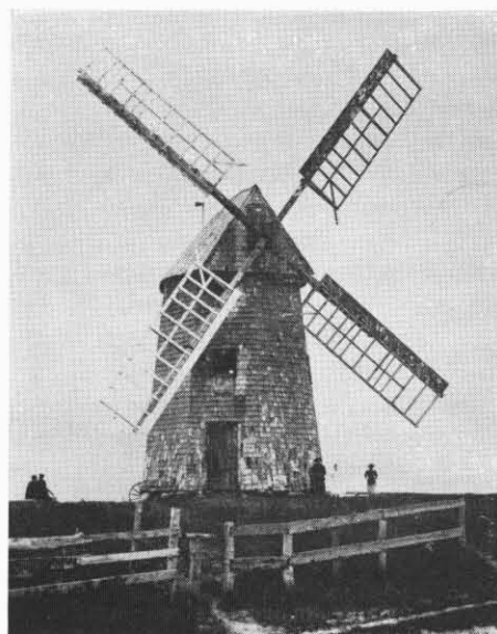
The only movable parts of the tower mill are its sails, also called arms.
