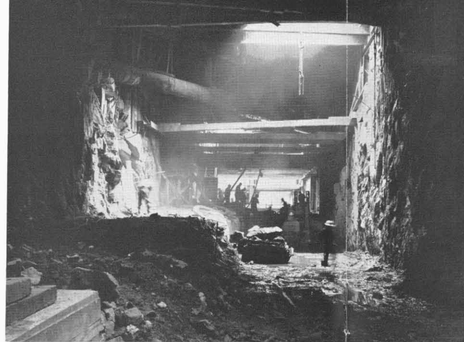
Planting dynamite calls for trained technicians, but in their hands the explosive is a useful tool for heavy jobs, such as pushing this subway through rock at Long Island City, New York.
