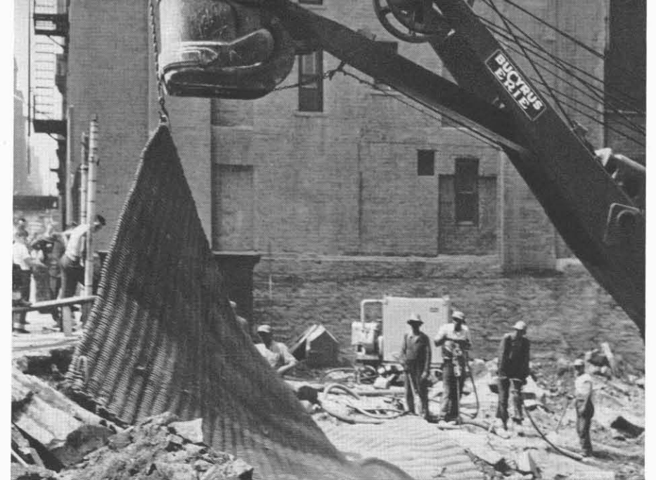
Flying debris is prevented by covering the blast site with tough, steel nets.
