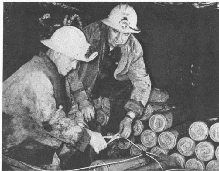
Planting dynamite calls for trained technicians, but in their hands the explosive is a useful tool for heavy jobs, such as pushing this subway through rock at Long Island City, New York.
