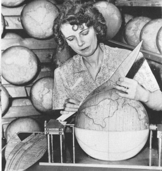
Map strips called "gores" align in exact relationship when pasted to a curved surface. The idea of gores is as old as map shown above, designed by a seventeenth-century map maker.
