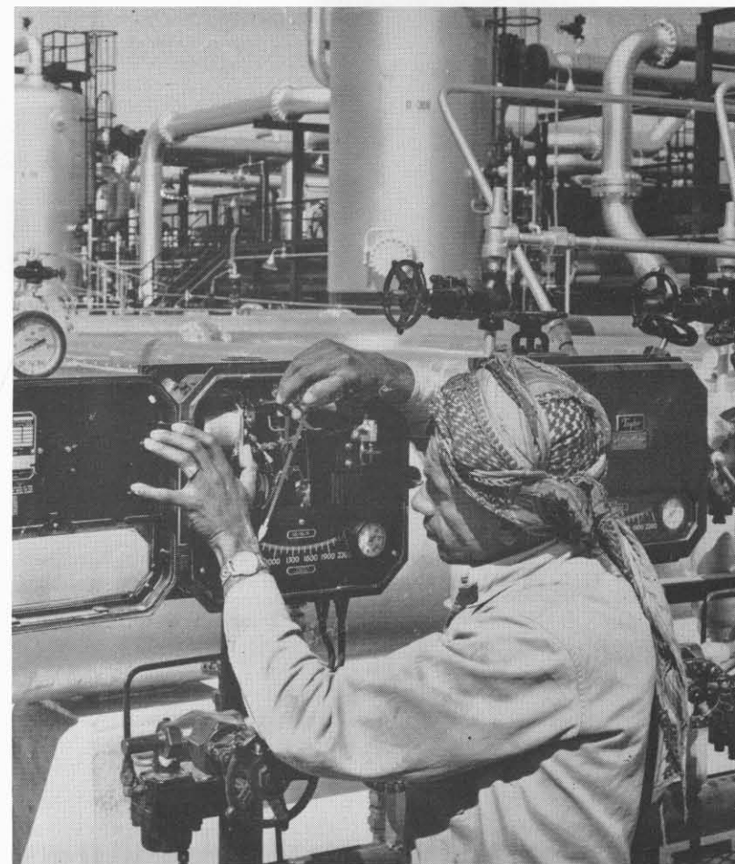
At 'Ain Dar Gas Injection Plant a technician adjusts a pressure controller in final stage of gas compression.
