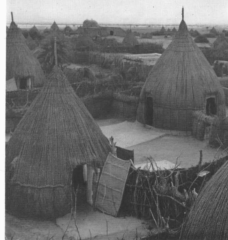
The conical "aushs" typical of the Jaizan coast are built of reed thatch and are architecturally unique in Saudi Arabia.
