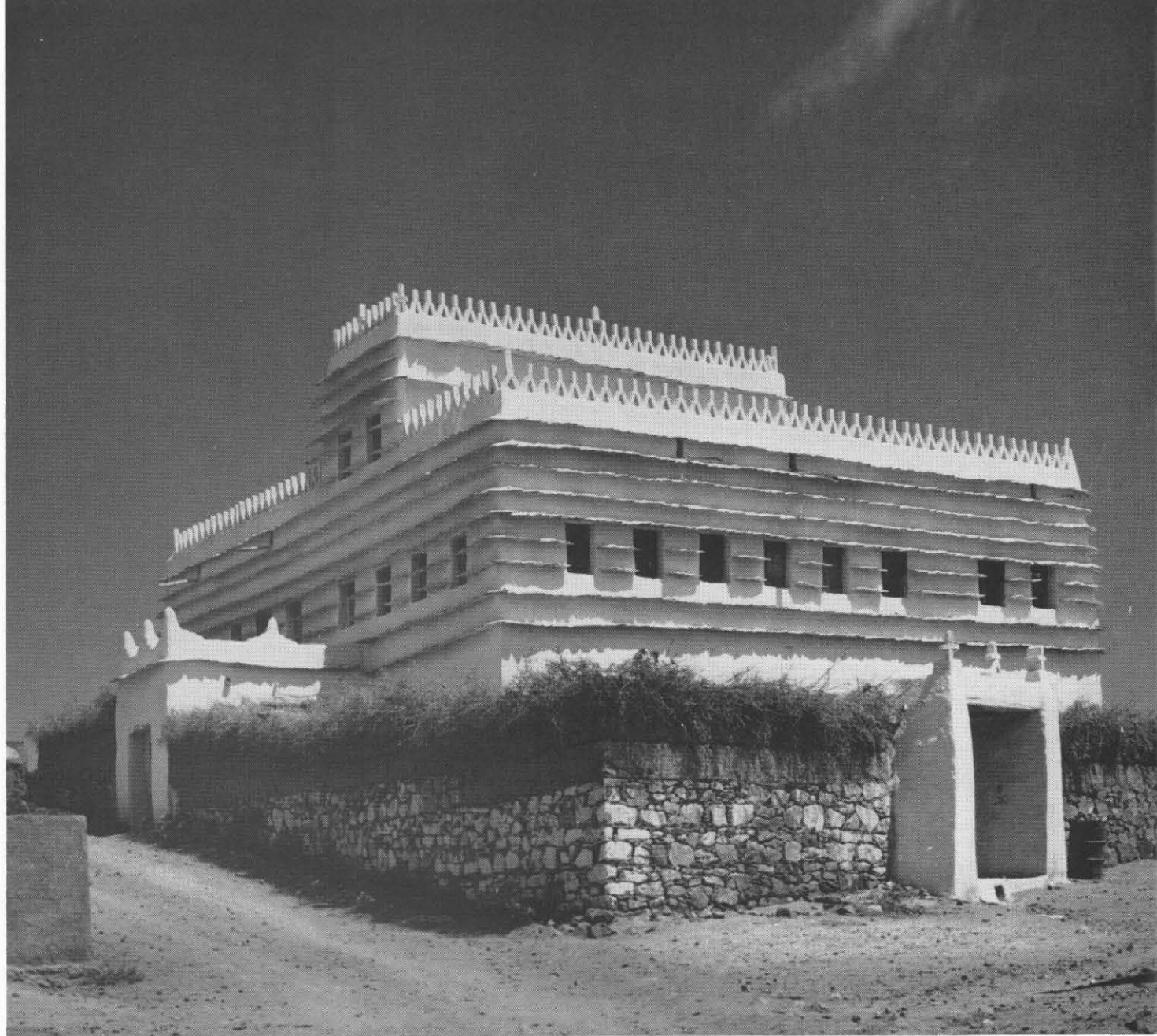
Clay brick houses in 'Asir's highlands are lined with slate to prevent rain from washing away facades.
