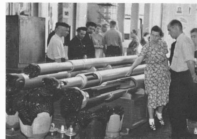
Moscow industrial fair, 1956, exhibited turbodrills driven by the high pressure of the drilling fluid.
