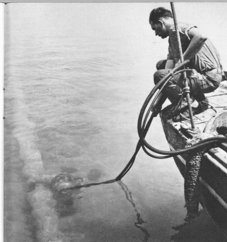
Diver checks submarine pipeline that carries crude oil from Saudi Arabia to Bahrain refinery. Aramco laid the first line in 1945 and another in 1952.
