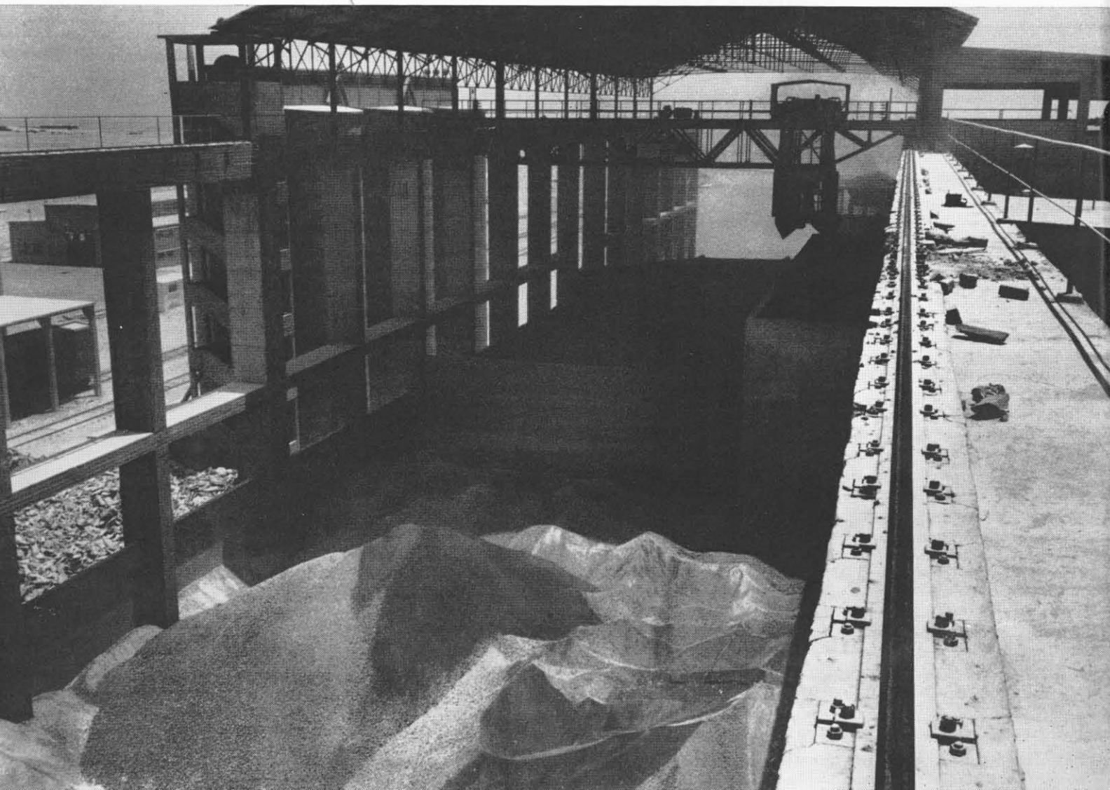
The vast raw materials storage hall of the Saudi Cement Company where crushed limestone, clay, iron ore and gypsum are piled before processing.
