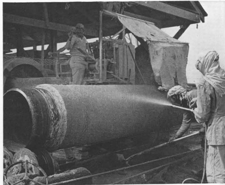
Saudi Arab contractor's workmen apply coating of cement to pipe that will form gathering system when Manifa offshore field goes on stream.
