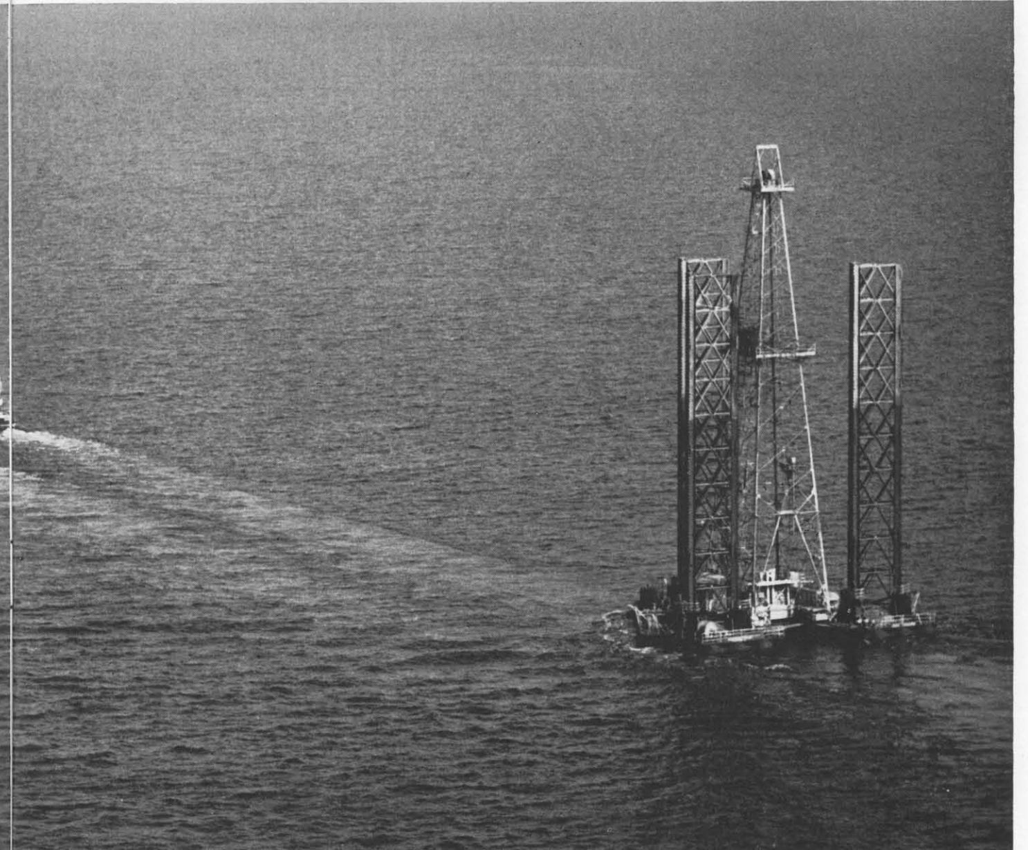
Aramco tugs tow drilling rig to Manifa in Persian Gulf. When rig is at well site, three legs, raised here, will be lowered to Gulf's floor.
