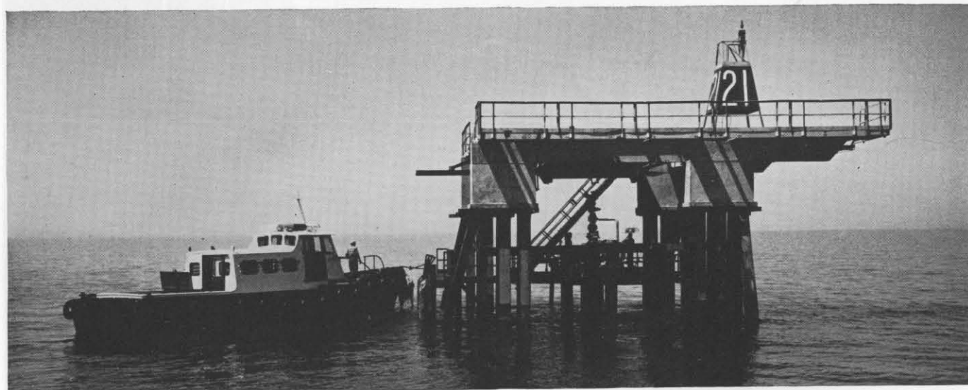
This completed offshore well with its Christmas tree platform is at Safaniya field but is similar to platforms that will be used at Manifa.
