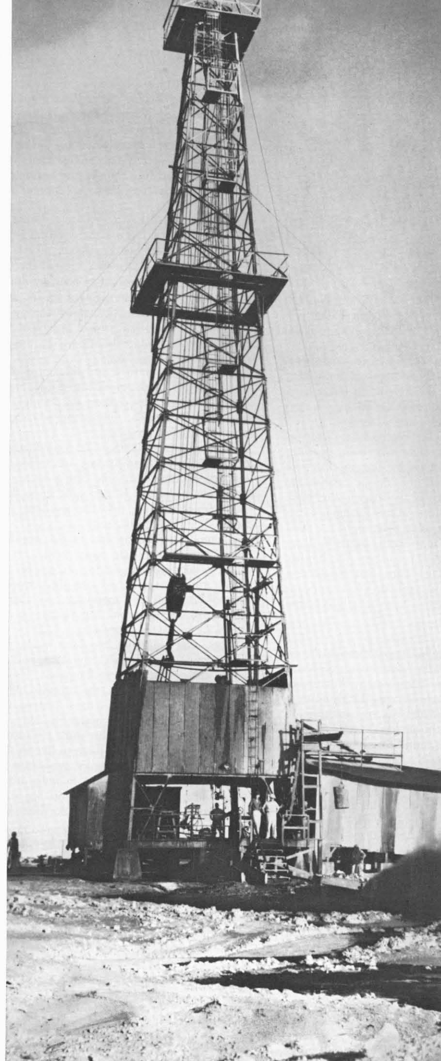
Drilling on Dammam No. 1, first oil well in Saudi Arabia, began in February 1935. Test flow made four months later when the well was down to 1,959 feet proved discouraging, but work was already underway on six more wells.
