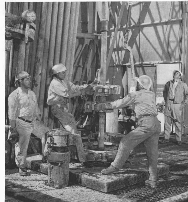
At bottom of the rig on the drilling floor, a crew of roughnecks works around the rotary table, which rotates drill pipe and bit like a carpenter's drill. At right is the tool pusher (drilling foreman).
