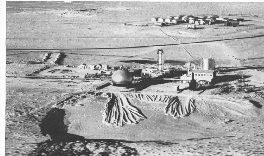
New gas-oil separator plant and stabilizer at Abu Hadriya processes crude oil by removing natural gas and corrosive hydrogen sulfide.
