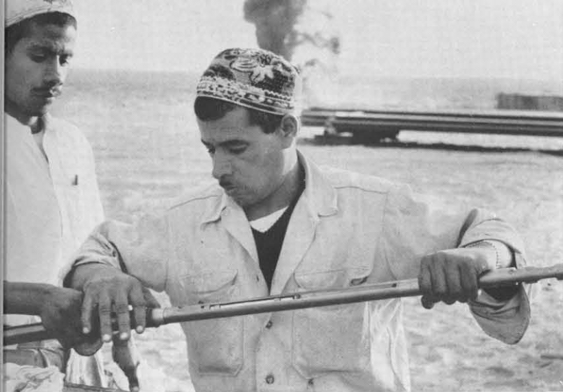
Field crew prepares to take pressure measurement deep in oil reservoir. Information is used at Dhahran to aid in predicting reservoir performance.
