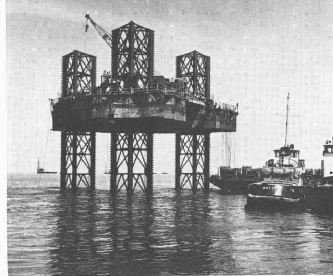
With her legs resting on floor of the Persian Gulf, AMDP-1 is being readied for installation of drilling rig on the platform. Barge 136 (below), popularly known as Queen Mary, works with AMDP-1 at Manifa field. After nearly 10 years' service Queen Mary was converted in 1963 to pipelaying and heavy-lift barge.
