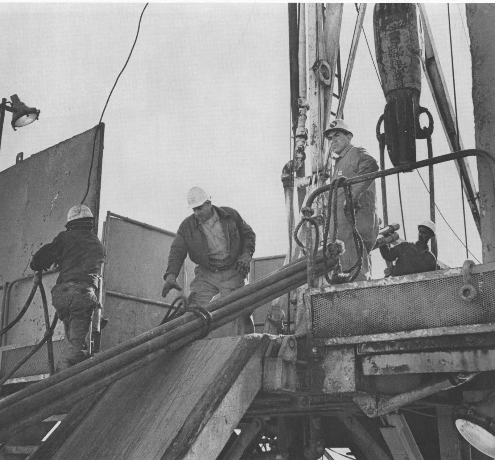
At the beginning of a twelve hour shift at an Abqaiq field workover rig, Kishi supervises the lifting of a string from pipe rack.
