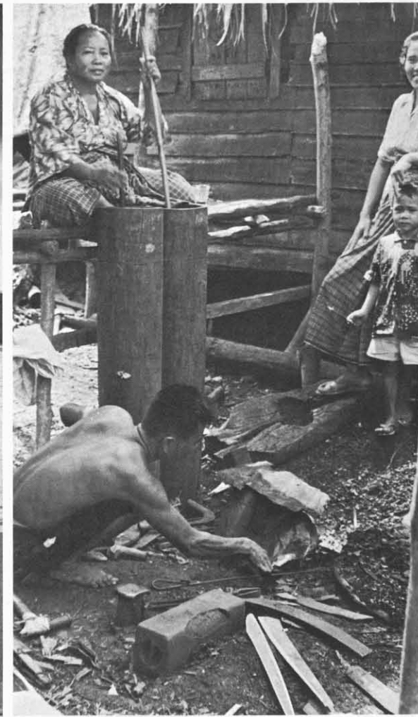
Blacksmith in Bongoa shapes swords and knives in homemade forge.
