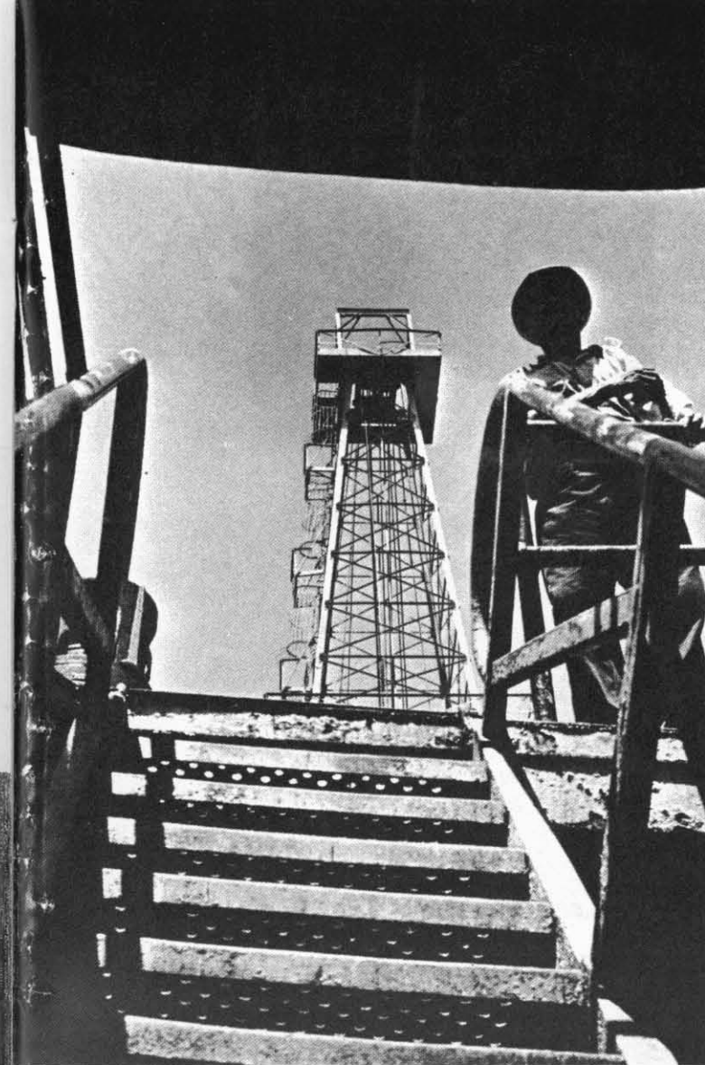
Drilling derrick on mobile drilling platform, seen through companionway of drilling tender, remains erect when platform is moved to new location.
