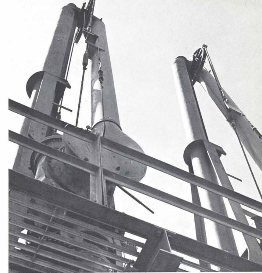
Once underway, work on the huge mooring dolphins, upper left, the 60-foot-long legs, lower left, and the Chiksan loading arms moved swiftly to completion.
