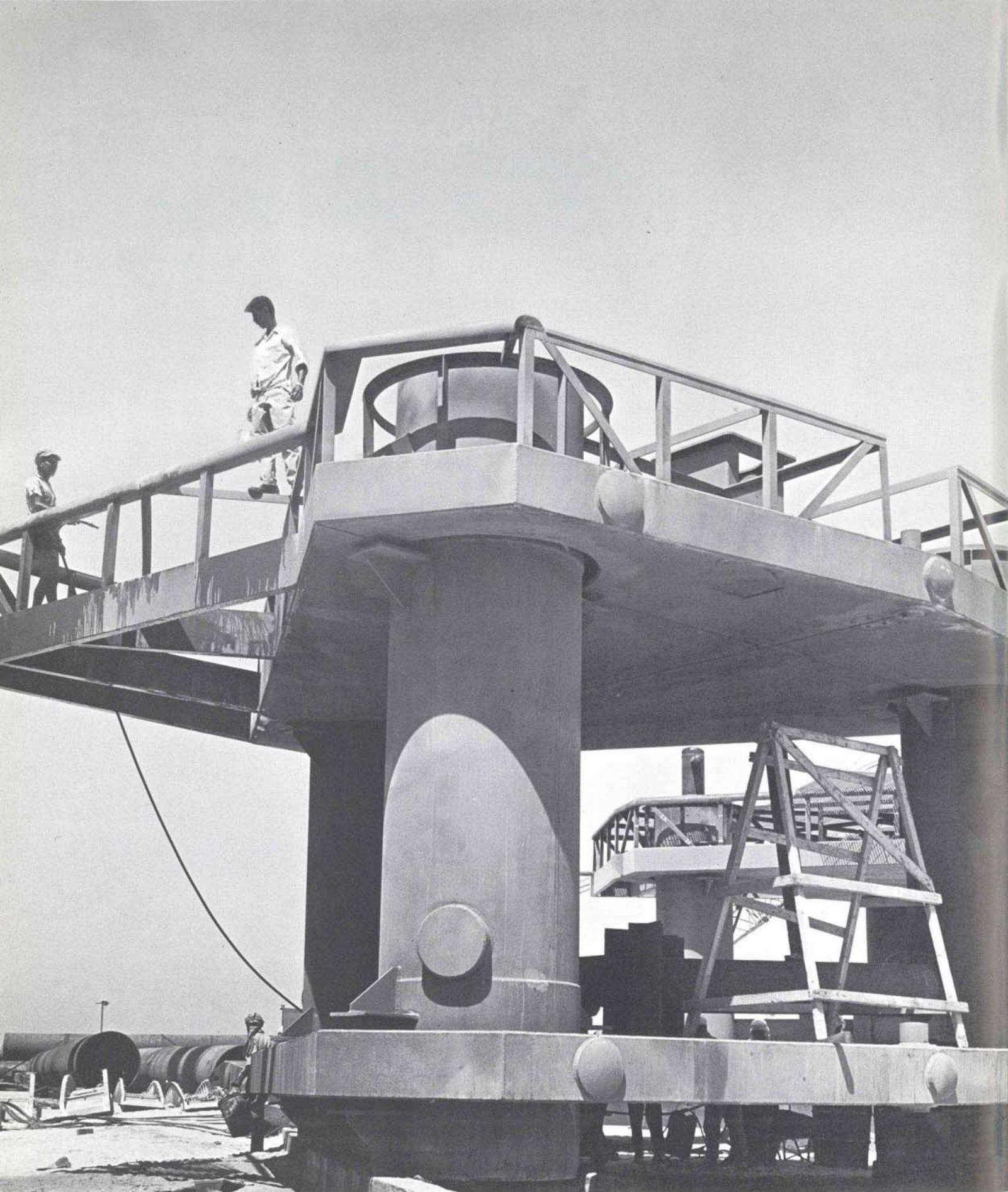
At the DeLong-Hersent-Kanoo Shipyard on Bahrain welders put finishing touches on top structure of one of eight breasting dolphins manufactured for Sea Island No. One.
