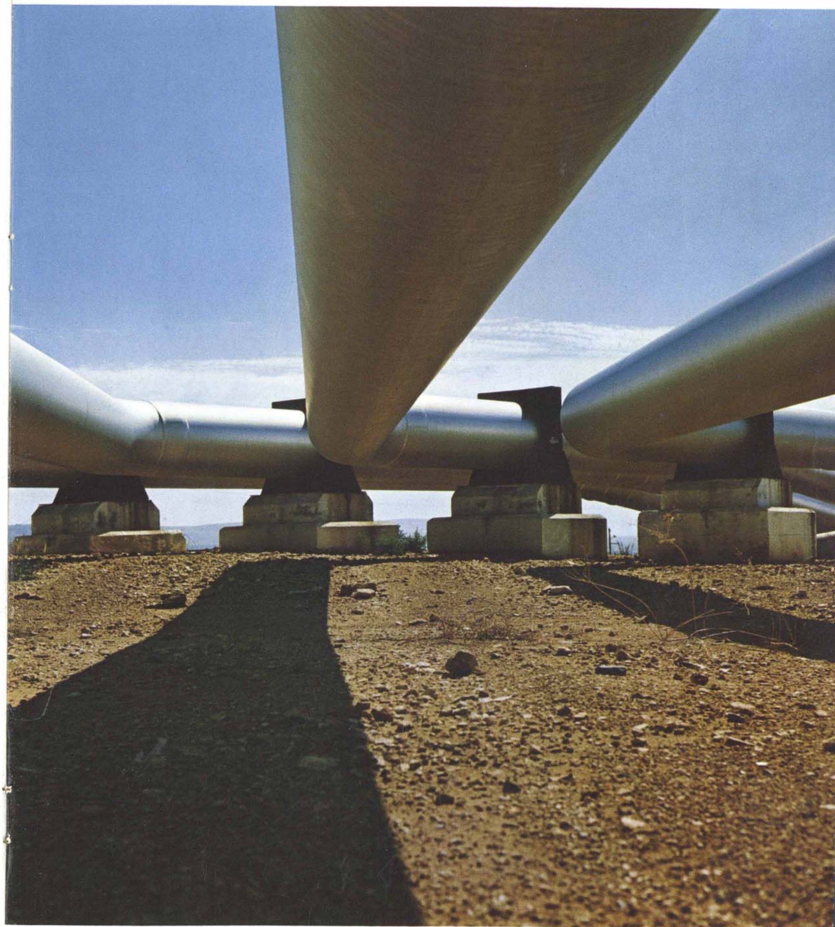
By force of gravity four mighty pipes feed the underwater lines at the end of which rubber hoses are coupled to the tanker's manifold; an 80,000-DWT supertanker can be loaded in about 10 hours.
