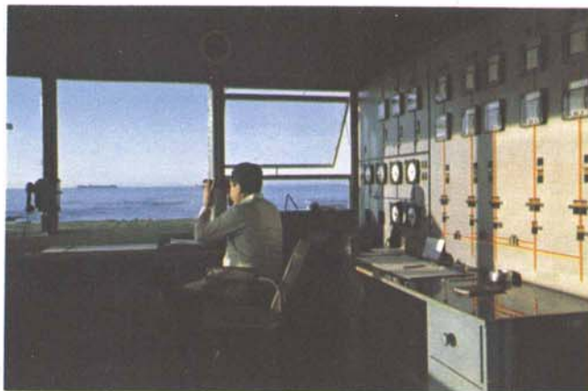
Shore control station operator regulates the flow of oil from tank farm to ships.
