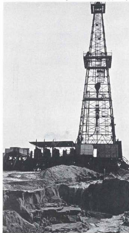
A rig with, left, draw works, mud pumps and diesel engines.
