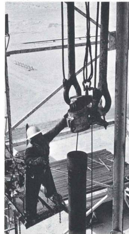
Guiding "elevator" as joints of casing are run into hole.
