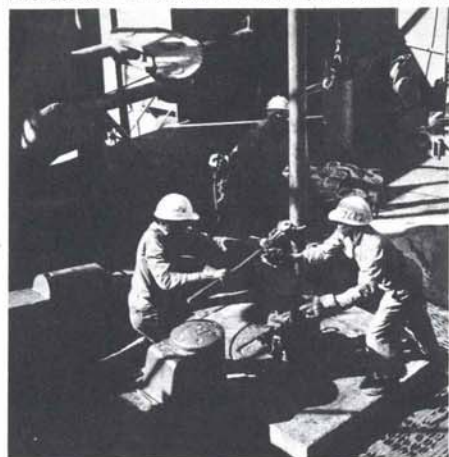
Aramco drilling team joins drill pipe at Abu Hadriyah.
