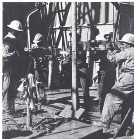
Drilling mud spurts from well as crewmen pull out pipe.
