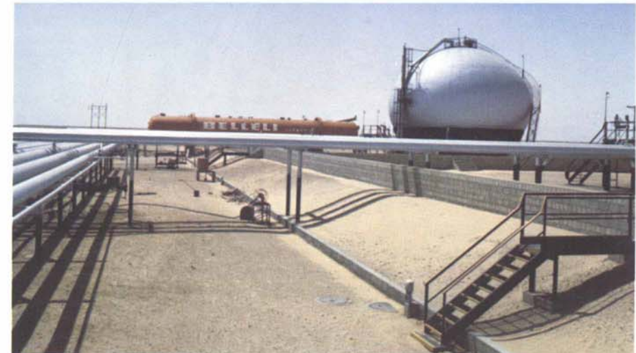
Installed and completed, the traps, center, and the spheroid, right, separate gas from oil by reducing pressure in stages.
