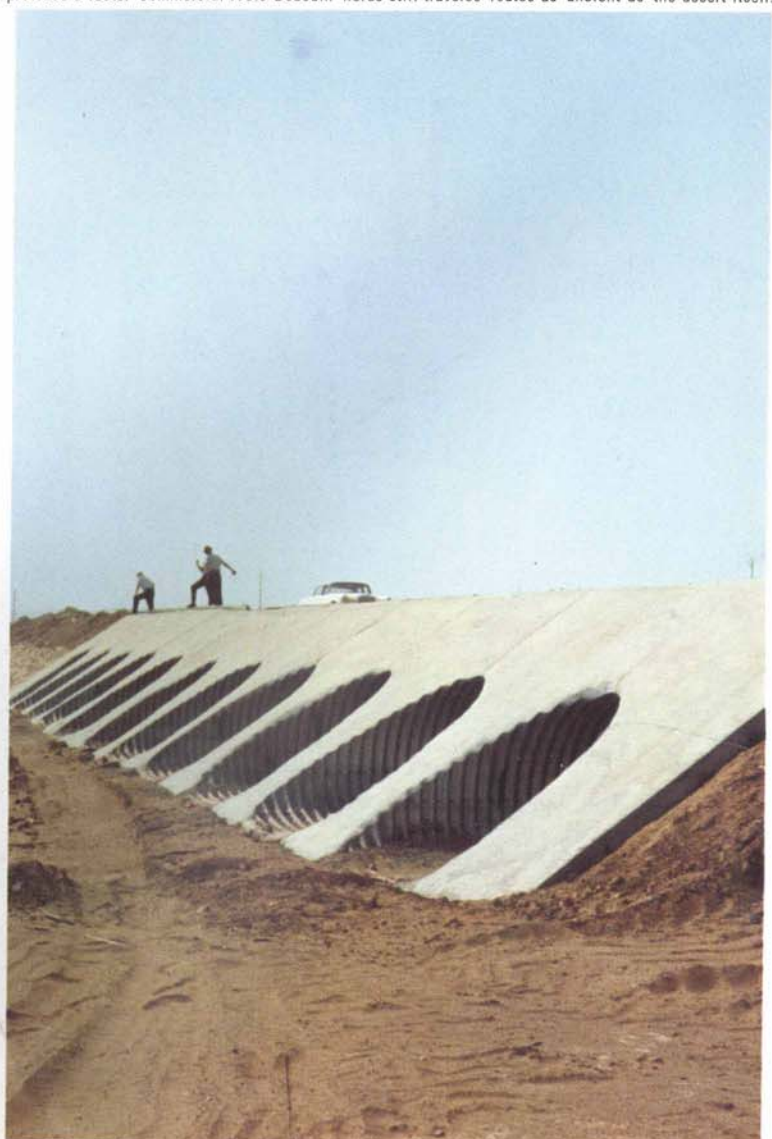
To cope with the country's rare but fierce floods builders had to install culverts in dry river beds.
