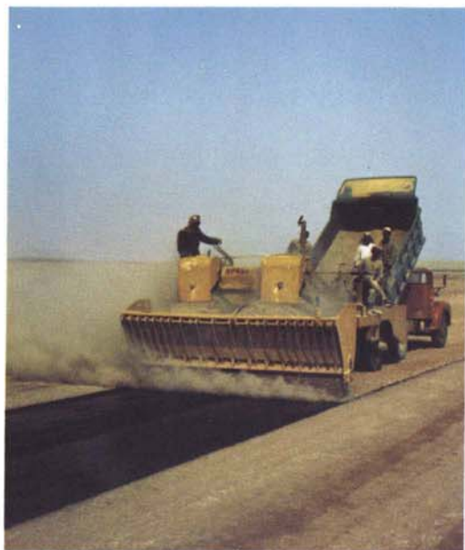
Crushed rock and second coat of asphalt make up first armor coat.
