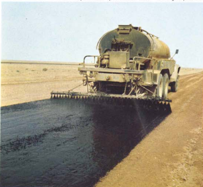
Nearing the final stages of construction builders spray asphalt over four inches of crushed rock.
