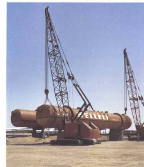
Two cranes lower the 175-ton cylinder down onto its foundations.
