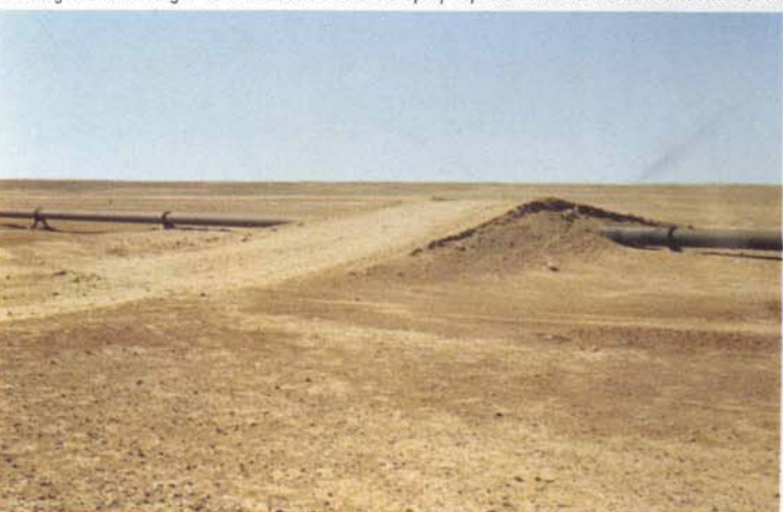
To allow animals to cross the pipeline camel crossings have been built at regular intervals.
