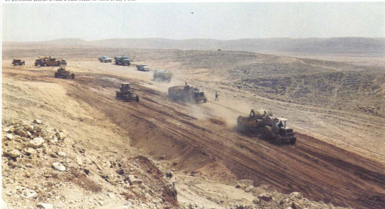
Earth-movers, bulldozers and motor graders all play noisy and spectacular roles in leveling hills, filling depressions and straightening potentially dangerous curves west of Badanah Pump Station.
