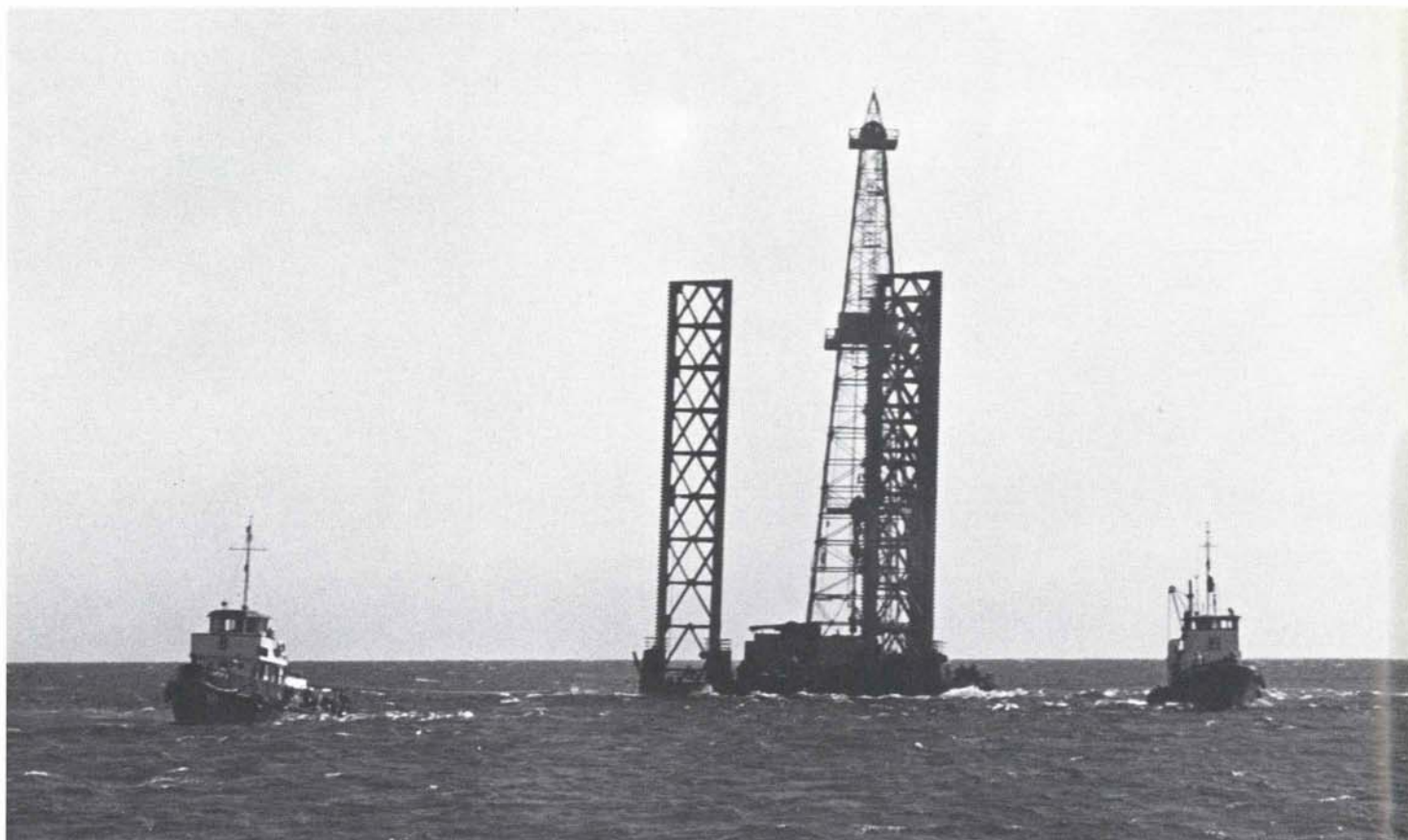
Aramco tugboats Qatif 8, Dammam 14 and Qatif 7 tow Drilling Platform No. 1 to a new job site about 20 kilometers offshore in the Arabian Gulf near al Jubail. During the move the drilling
