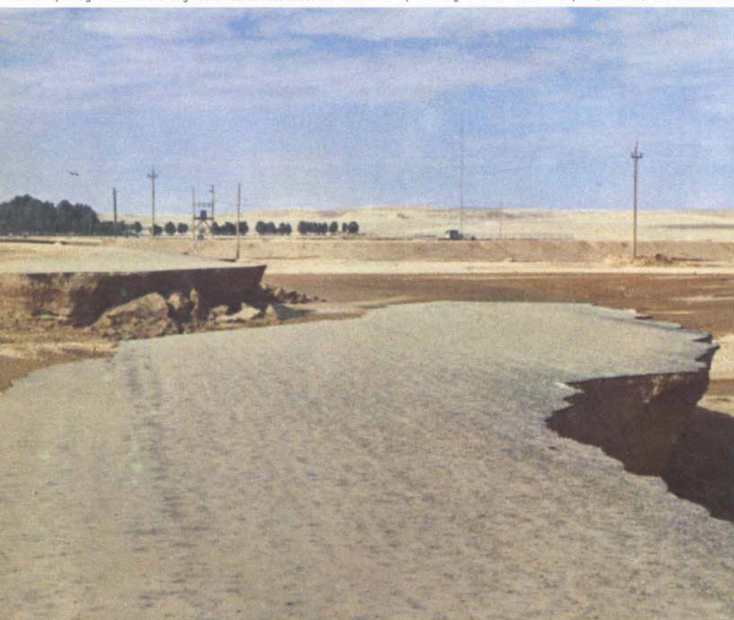
As the flood receded Tapline began to assess the damage and found that great sections of the newly completed road had been destroyed.
