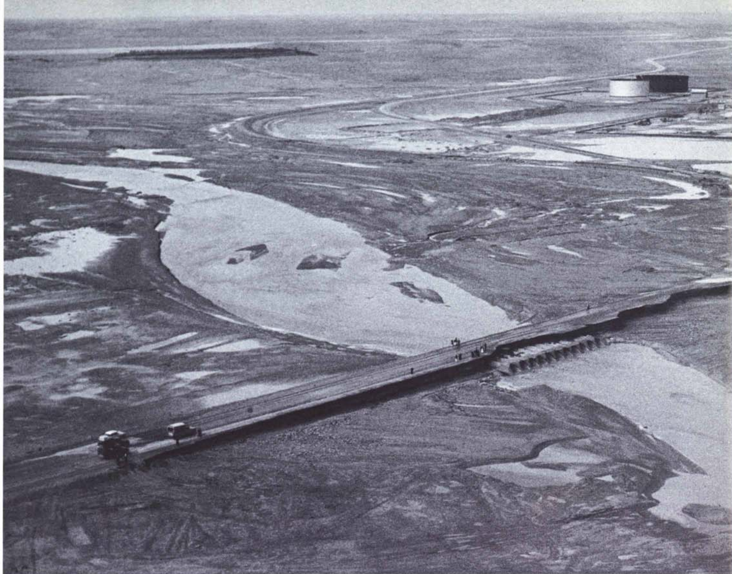
To be sure flash floods could not damage the new road Tapline bridged the Wadi Badanah with 11 culverts big enough to cope with 735 million gallons of water an hour, yet by mid morning a torrent of water 14 feet deep was spilling across the road.
