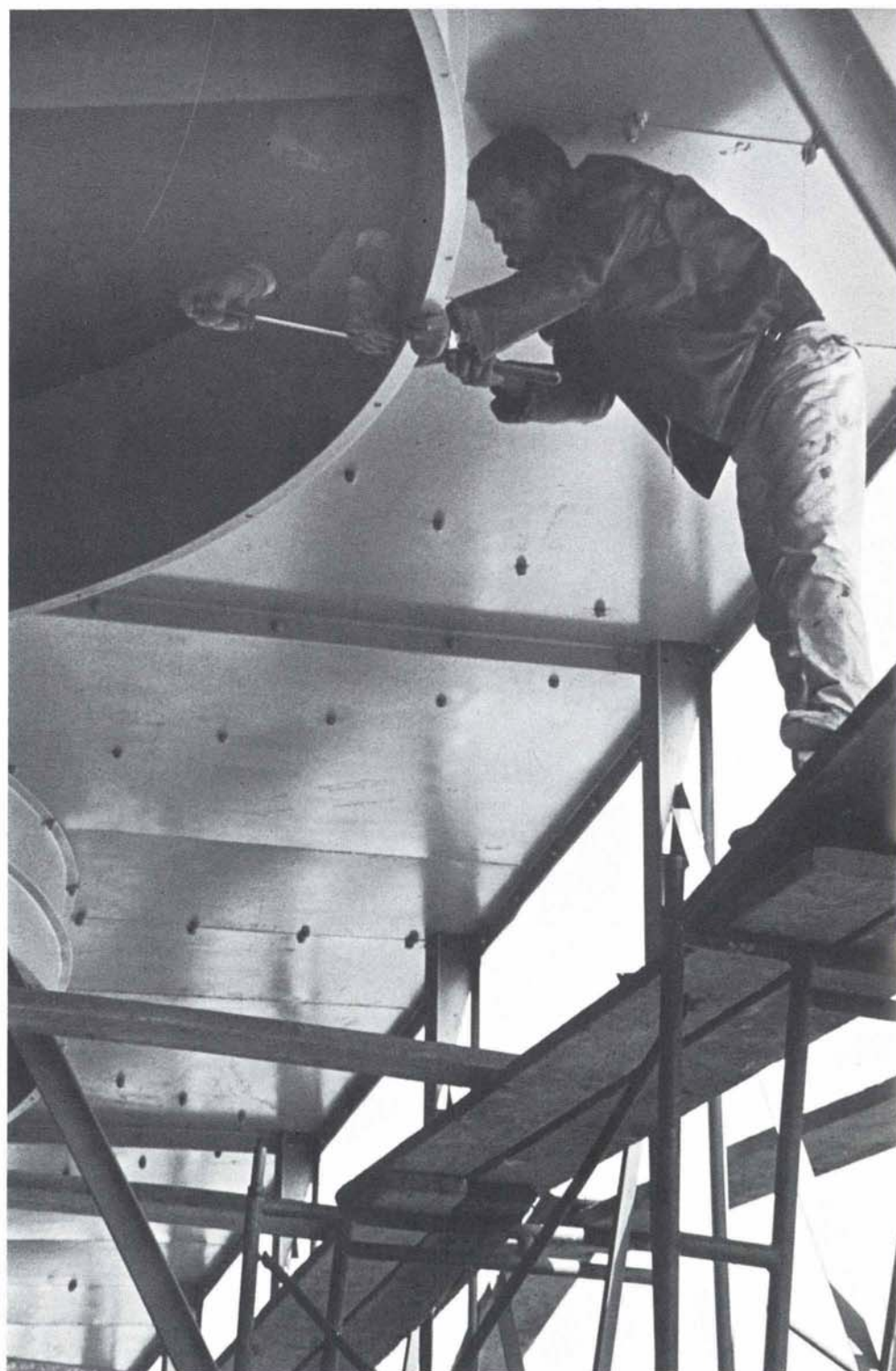
Iron workers in the Abqaiq industrial area prepare to install a shroud around an air cooler fan for a new stabilizer.
