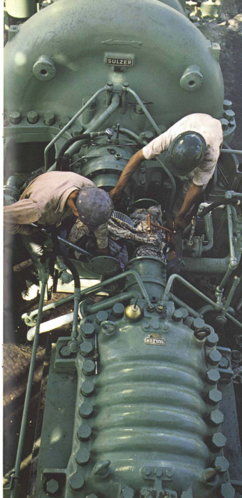
At Abqaiq's power plant, machinists install a new compressor.
