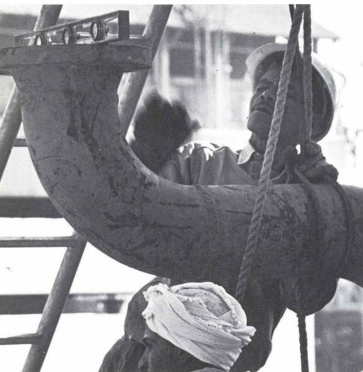
pipefitter adjusts a process pipe going into the new crude topping unit at Ras Tanura refinery.
