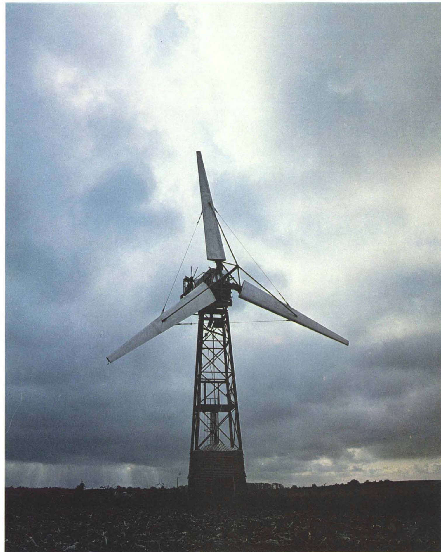
At Aldborough Manor in Yorkshire, Sir Henry Lawson-Tancred is experimenting with a 56-foot diameter "aerogenerator" able to produce 100 kilowatts of power at 30 mph.
