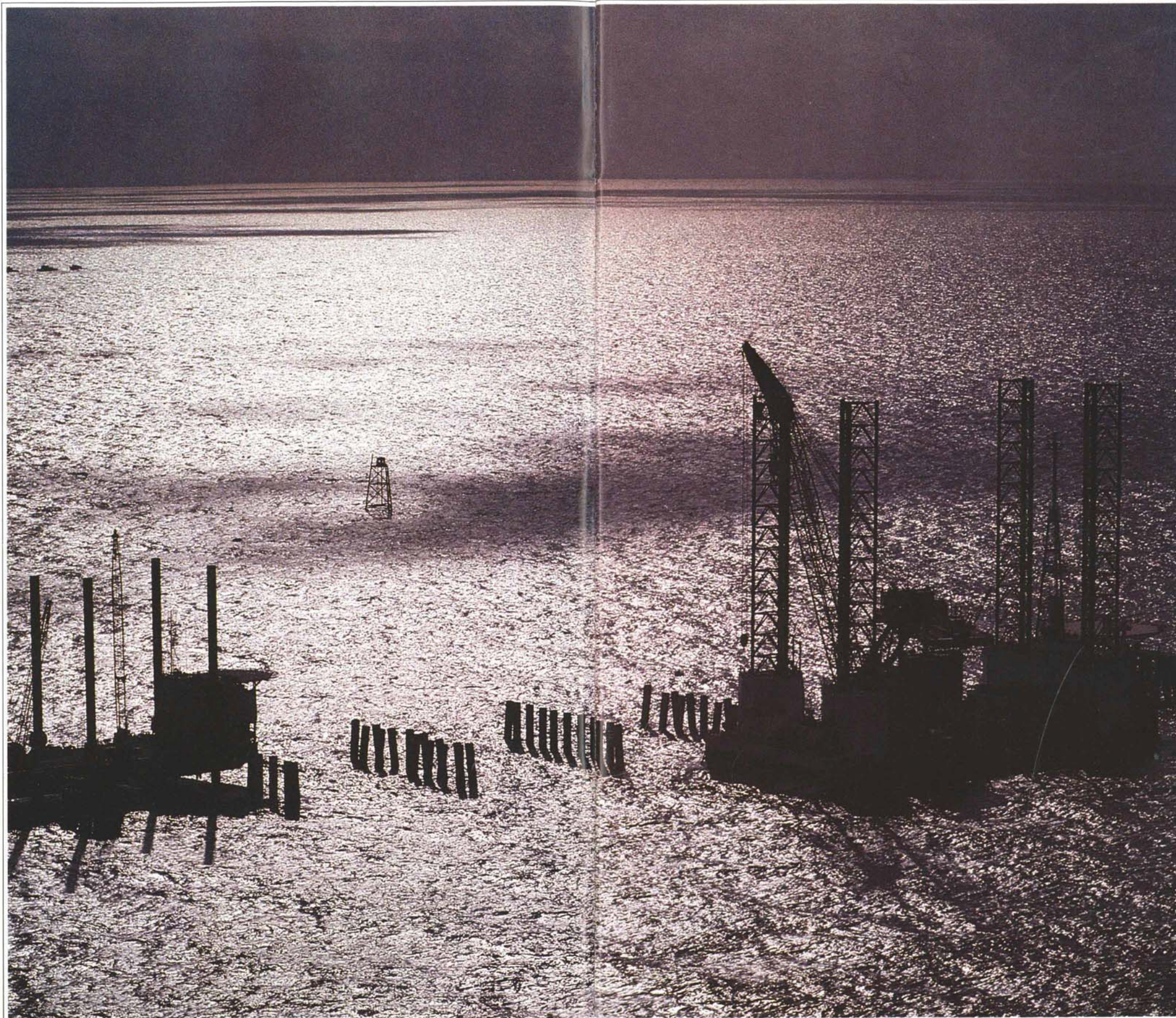
Above, the new computerized container terminal at Dammam, and right, under construction and complete, the 10-kilometer-long pier (six miles) carrying pipes to the offshore gas loading terminal at Ju'aymah.
