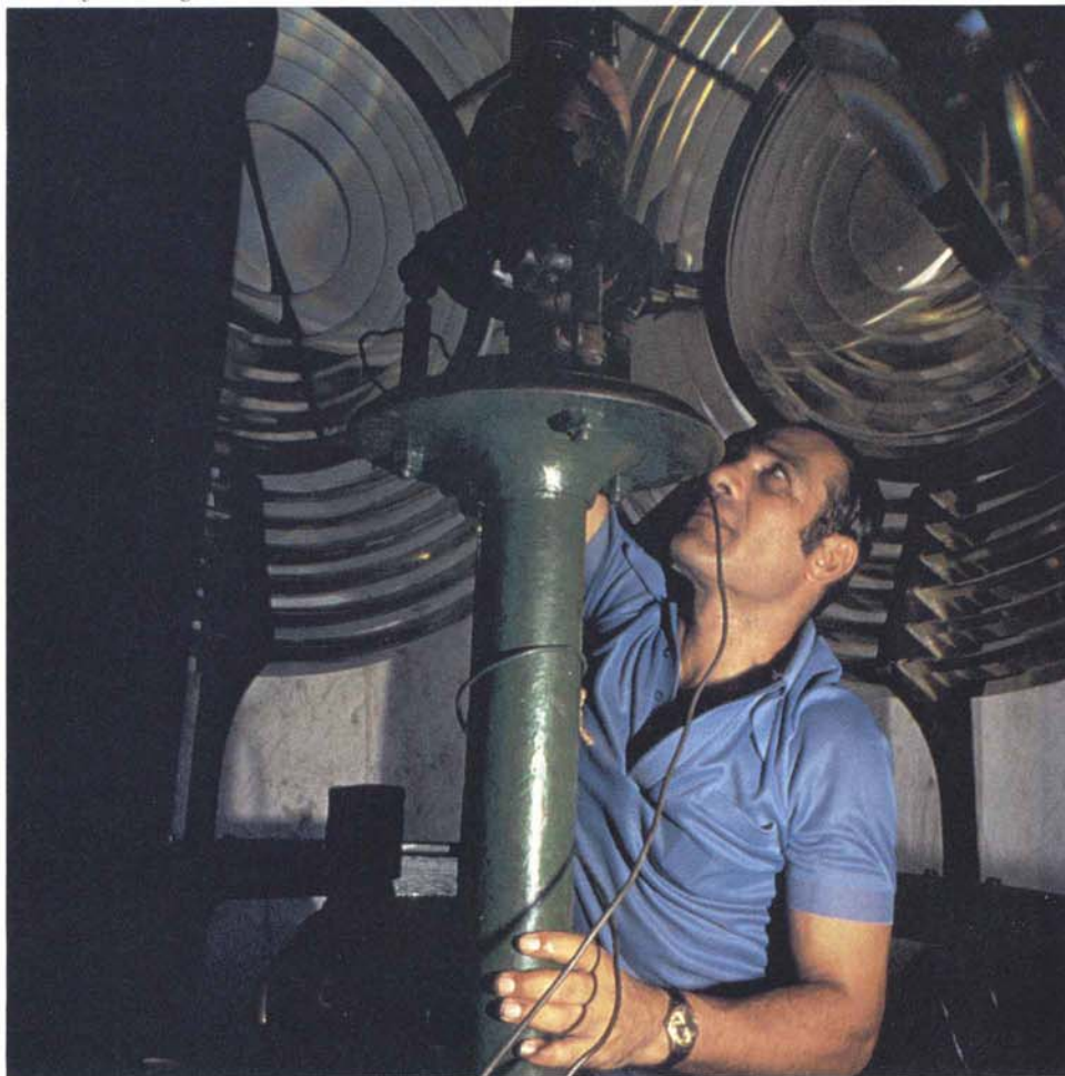
Captain Harga lights the great gas mantles of the al-Ikhwan lighthouse, a masterpiece of 19th century technology that includes a fresnel lens capable of magnifying light 200 times and flashing a beam visible 30 kilometers away.
