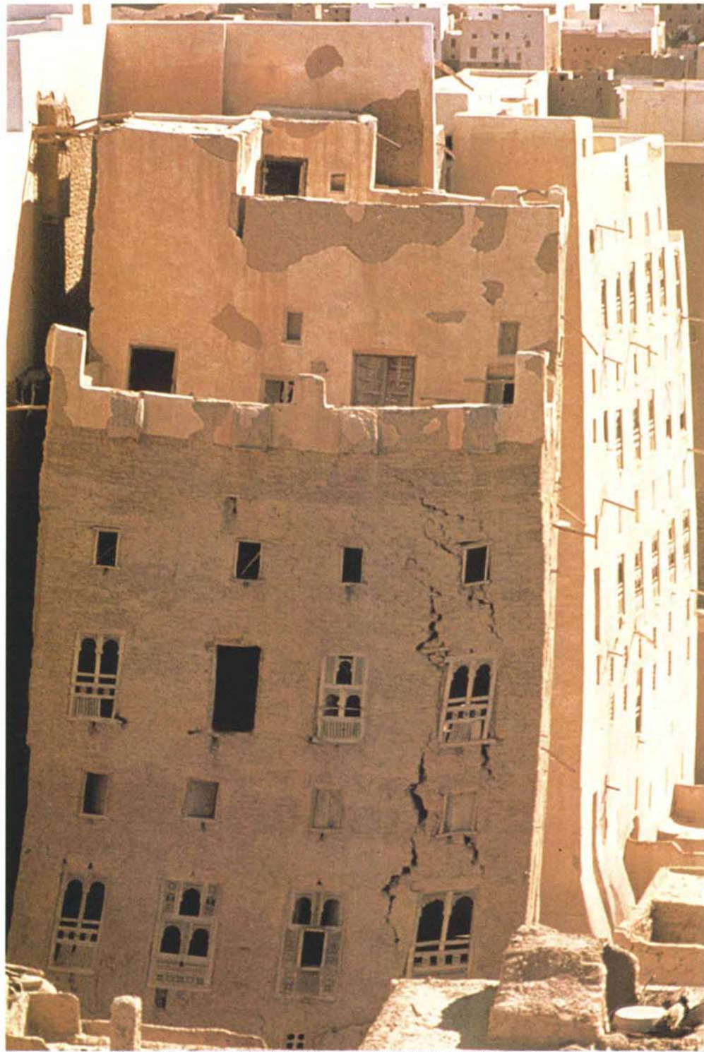
Huge cracks quickly appear in mud-brick buildings unprotected by regular coatings of waterproof plaster.
