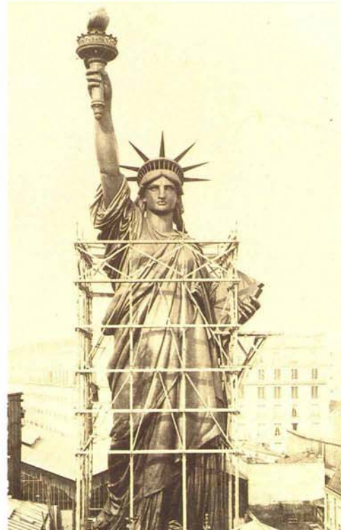
Liberty's hand, above, and head, opposite page, take shape in Galet and Gauthier's Paris workshop, while below, her body rises slowly around the iron skeleton designed by Eiffel.
