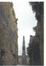
This carved rock needle at Saone, left standing when the moat was hewn from the mountain rock, supported a narrow wooden bridge that led to one of the castle's two entrances.
