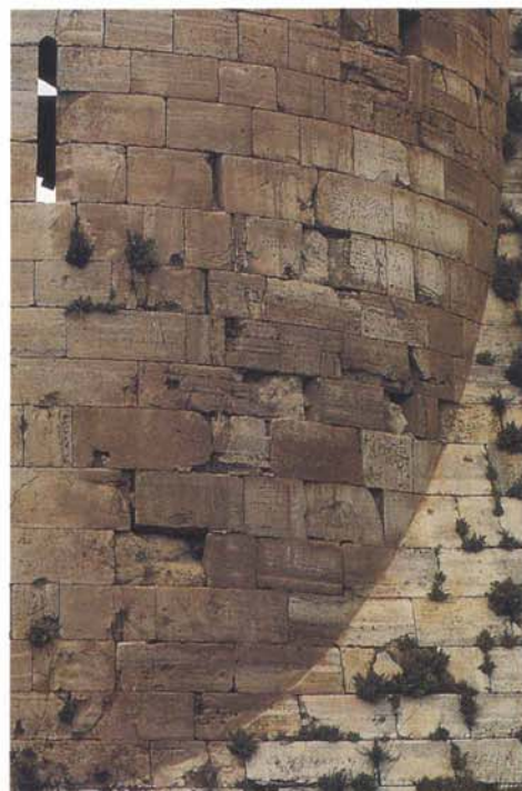
At the Krak des Chevaliers, a cylindrical tower meets the sloping talus in a complex curving fold. No two stones meet at this join, however. Instead, individual blocks—no two alike—were carved to bridge the transition without giving attackers a foothold.
