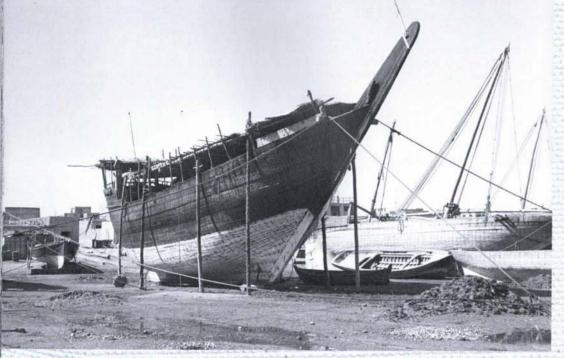
Dhows were fashioned by master builders. Shown left is a typical Kuwaiti boom under construction on the waterfront. Below: The Triumph joined larger baggalas like this one for a hull cleaning by the crew at Kwale Island, off today's Tanzania, before picking up its cargo of mangrove poles a little farther
