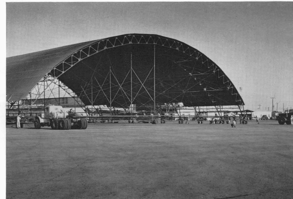
To make room for construction of the new terminal building at Dhahran International Airport, a hangar was "put on wheels" and towed by truck to a different location a quarter-mile away.
