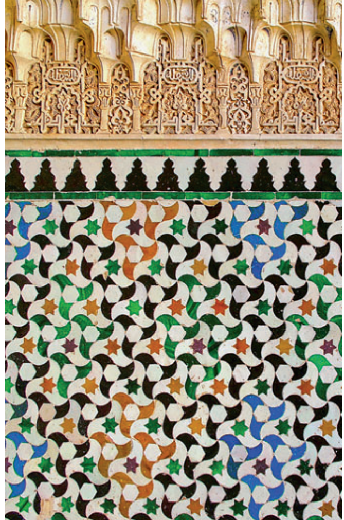
Multicolored tiles seem to swirl through space in this alicatado (cut-tile) pattern produced in the 14th century by Nasrid artisans on a wall of the Court of the Myrtles in the Alhambra palace in Granada, Spain. The Arabic root of the Spanish alicatado is al-qata , “the cut.”
