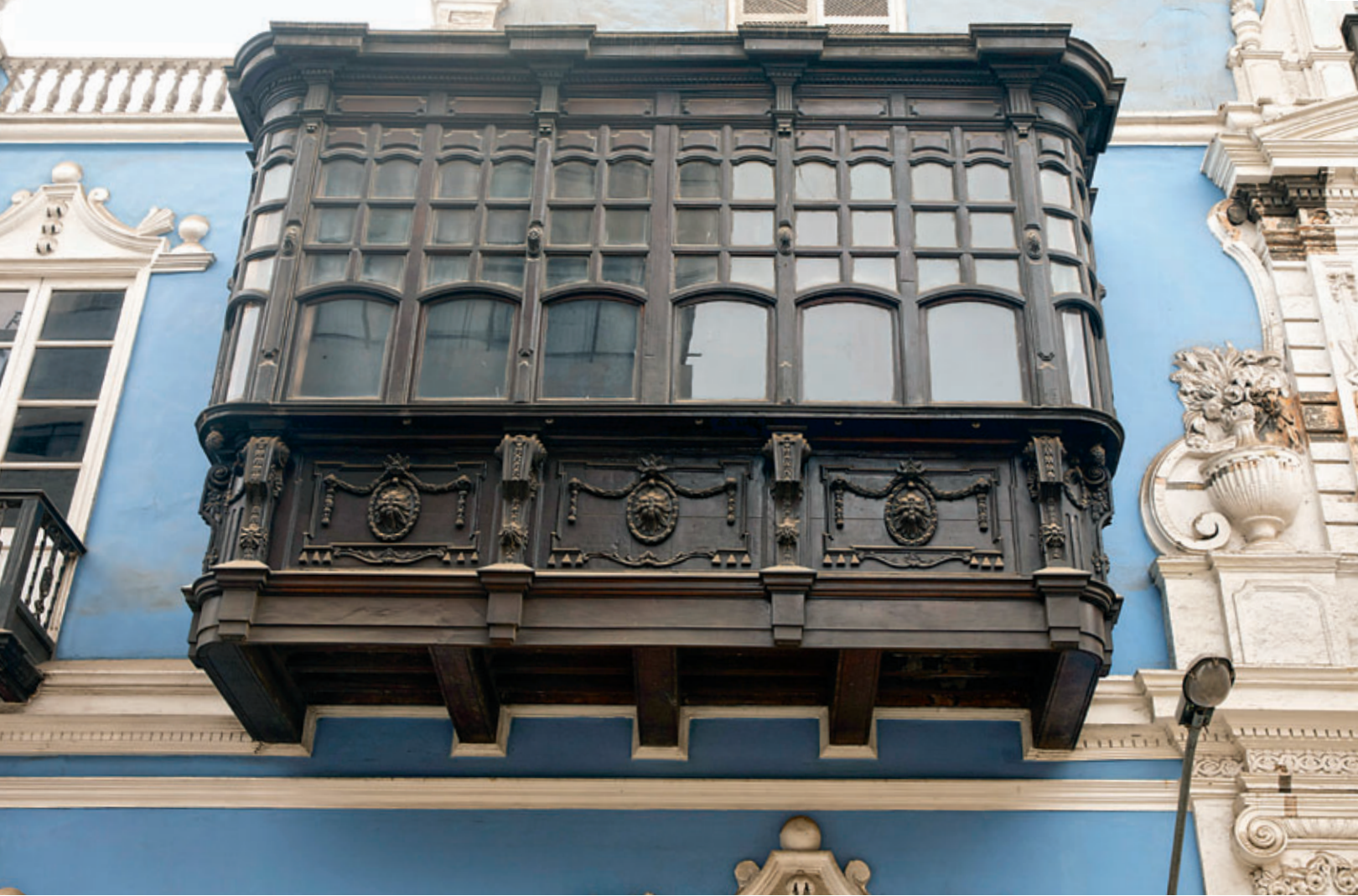
Built at the turn of the 19th century by a Spanish merchant and recently restored, the balconies along the facade of the Casa Osambela reflect an entirely European, neoclassical style. LOWER Along Jirón Ancash, a balcony reflects an eclectic 20th-century style. The interplay of similarities and differences in Lima's balconies led 20th-century Peruvian composer Luis Antonio Meza to describe them as "homogeneous and harmonic."
