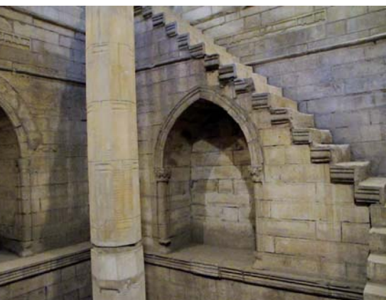
The sluice-gates of the Nilometer, built 108 years before the founding of Cairo, are the earliest known pointed arches in Egypt.
