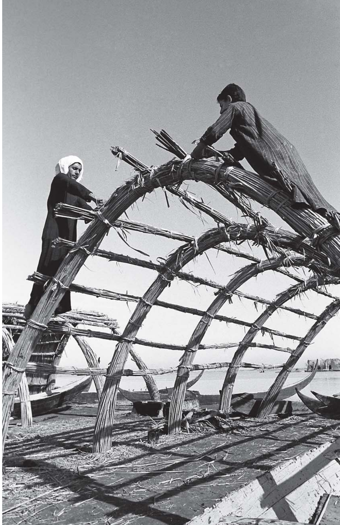
Men build a house from bundled reeds in the village of Al-Dubbon. After more horizontal bundles are added, it will be roofed with mats of split, plaited reeds that direct rainwater down the sides.
